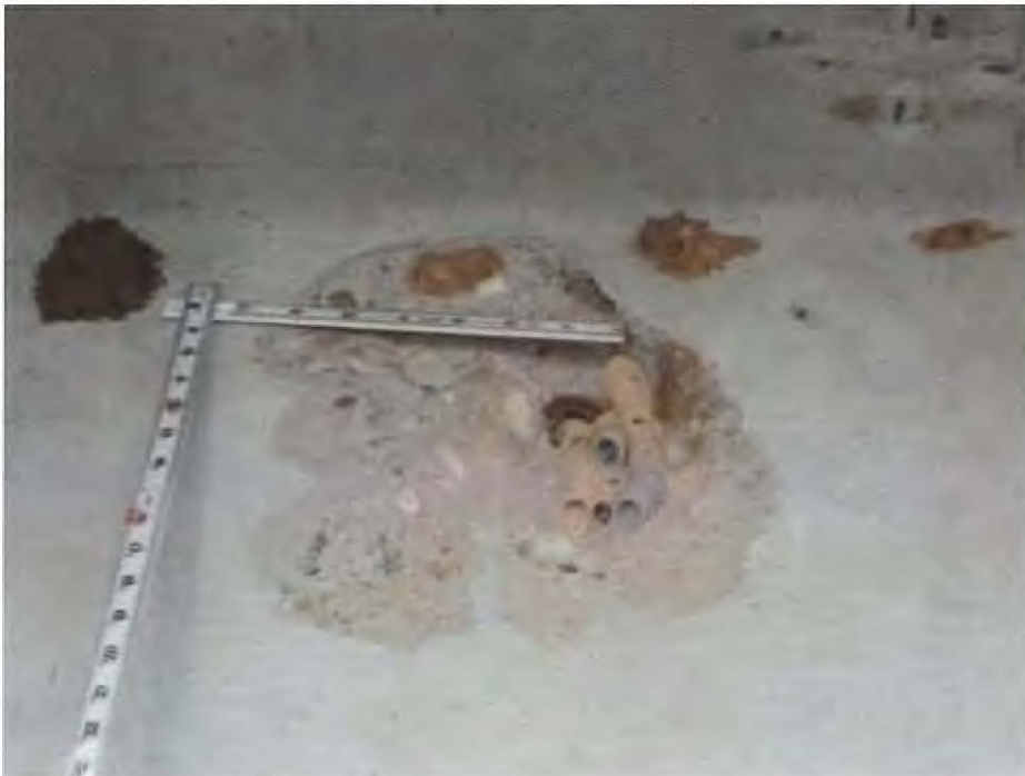
109 - Pre Opn Conc Girder/Beam
