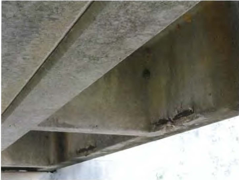
109 - Pre Opn Conc Girder/Beam
