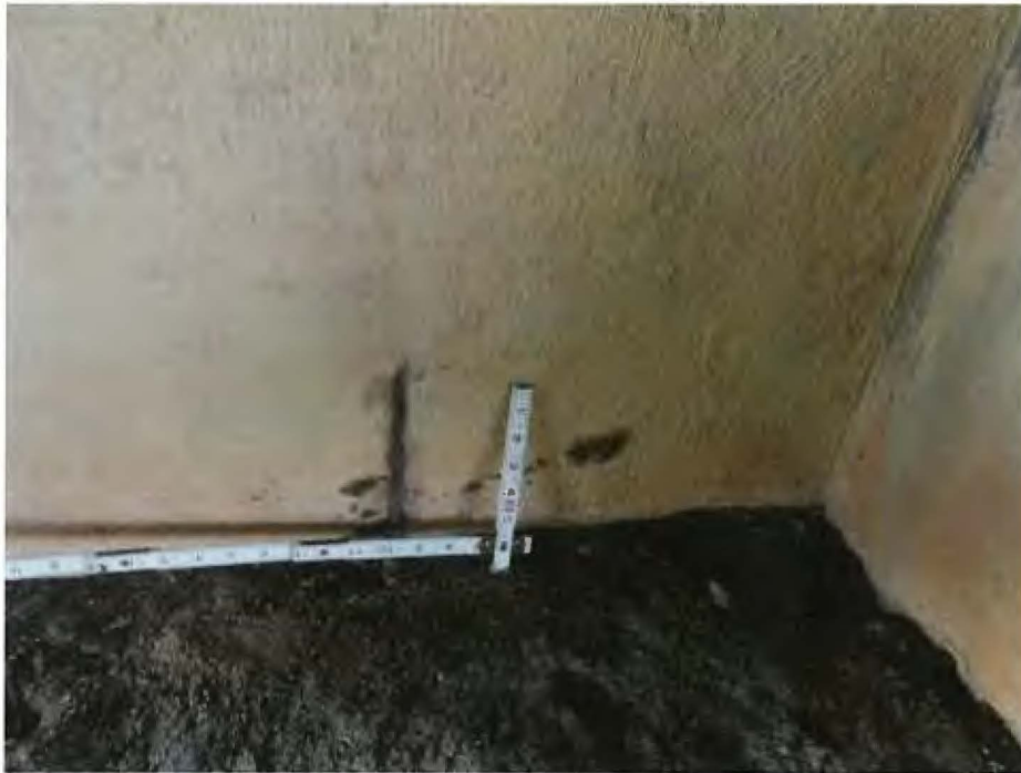
215 - Re Conc Abutment
