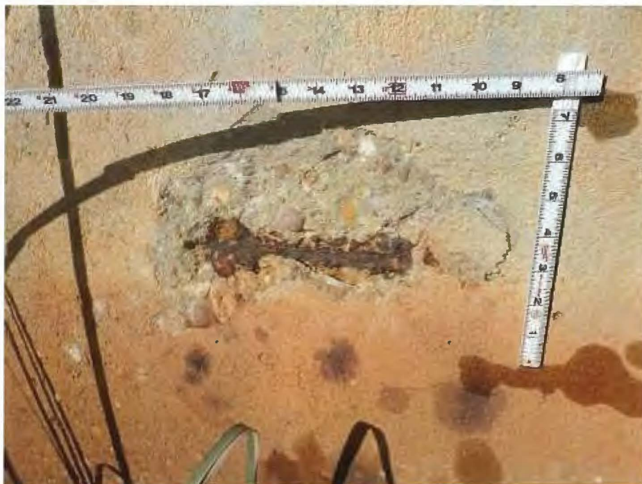
215 - Re Conc Abutment
