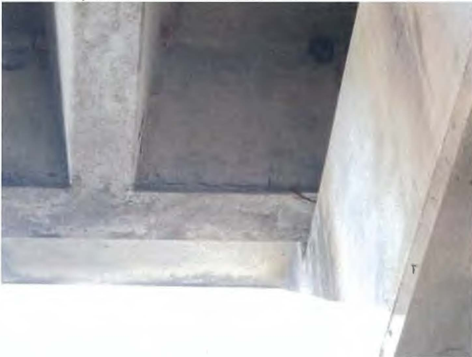
109 - Pre Opn Conc Girder/Beam
