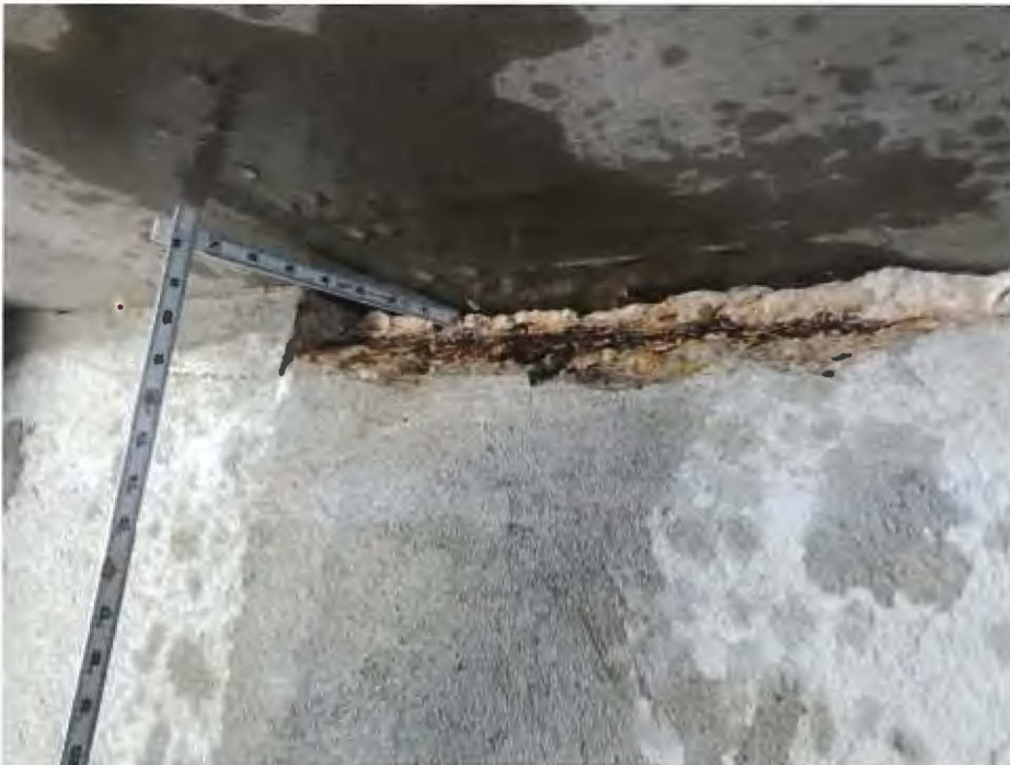
215 - Re Conc Abutment
