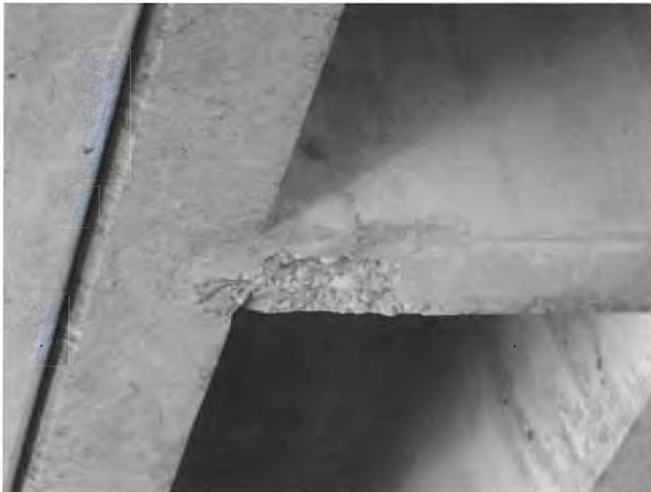
109 - Pre Opn Conc Girder/Beam
