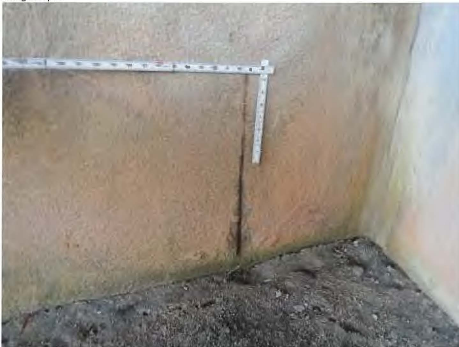
215 - Re Conc Abutment
