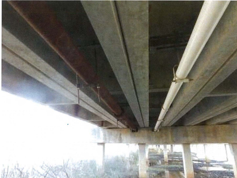
12 - Re Concrete Deck
