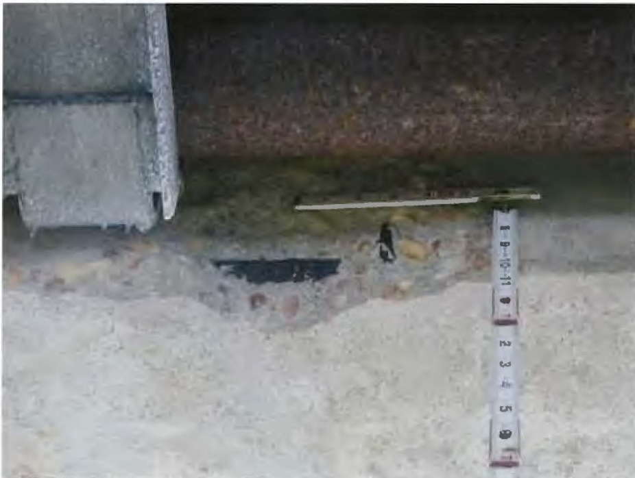
109 - Pre Opn Conc Girder/Beam
